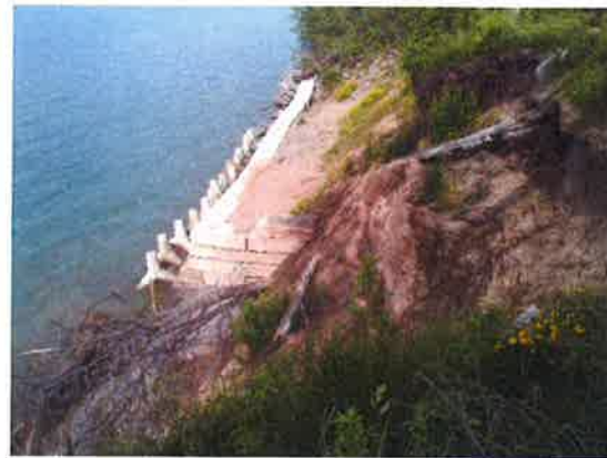
Example of isolated shoreline protection
