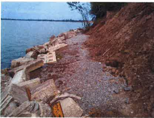
Poorly designed shore protection
