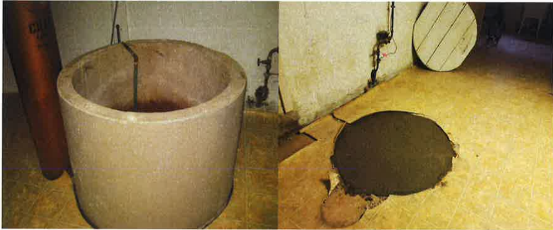
Figure 3. An example of a NPCA Water Well Decommissioning Project. Left photo shows an abandoned dug well in need of decommissioning and the right photo shows same dug well after decommissioning had been completed by a licensed well contractor.
