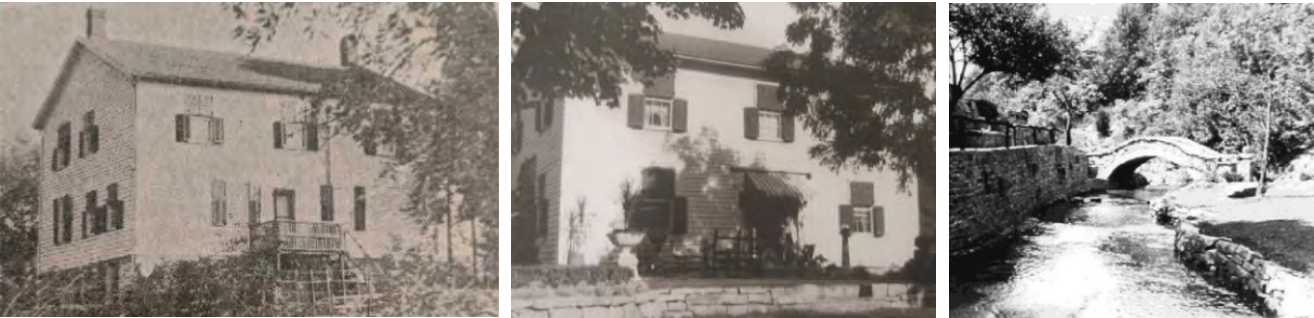
Historic views of rear and façade of the mill house ( both undated [ c. 1930s], courtesy of Nick Bogaert, 2025)
