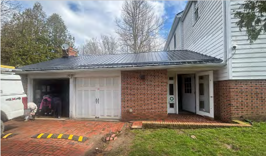
South Entrance Exterior
