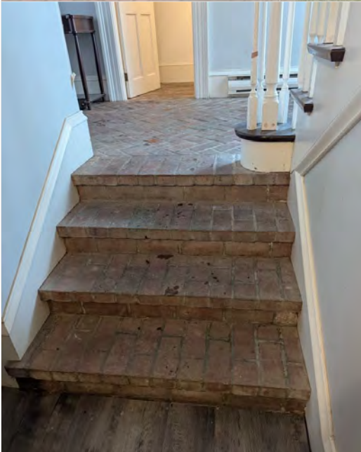
Front Door Landing Stairs to Basement
