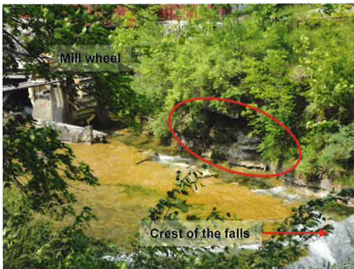
Some undercutting observed on the rock face (left bank downstream of the mill wheel)
