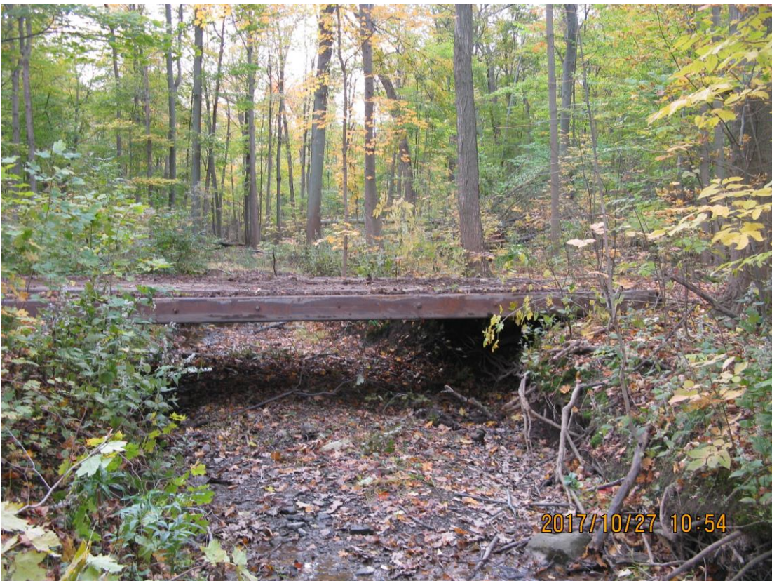
Figure 4: side view of the temporary portable bridge.
