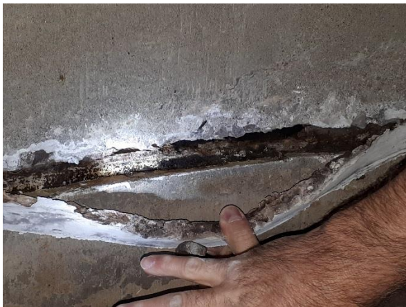
Existing joint sealant to be replaced.
