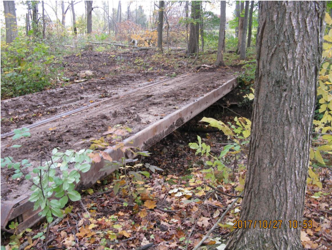
Figure 3: view of a temporary portable bridge used to gain access over a steep-bank stream.
