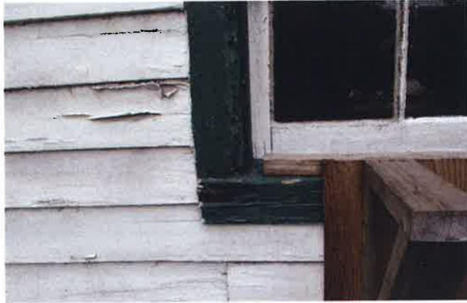
Rotted sill, no projection, south window, west wall (with air conditioner bracket)
