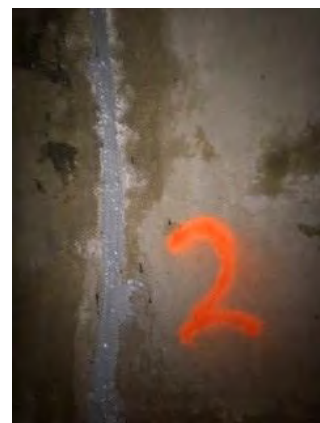
Picture 5. Newly sealed joint.
