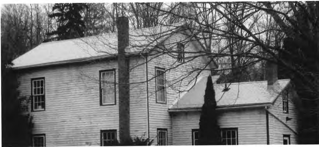
Metal roofing and aluminum troughs, cedar tree requiring removal
