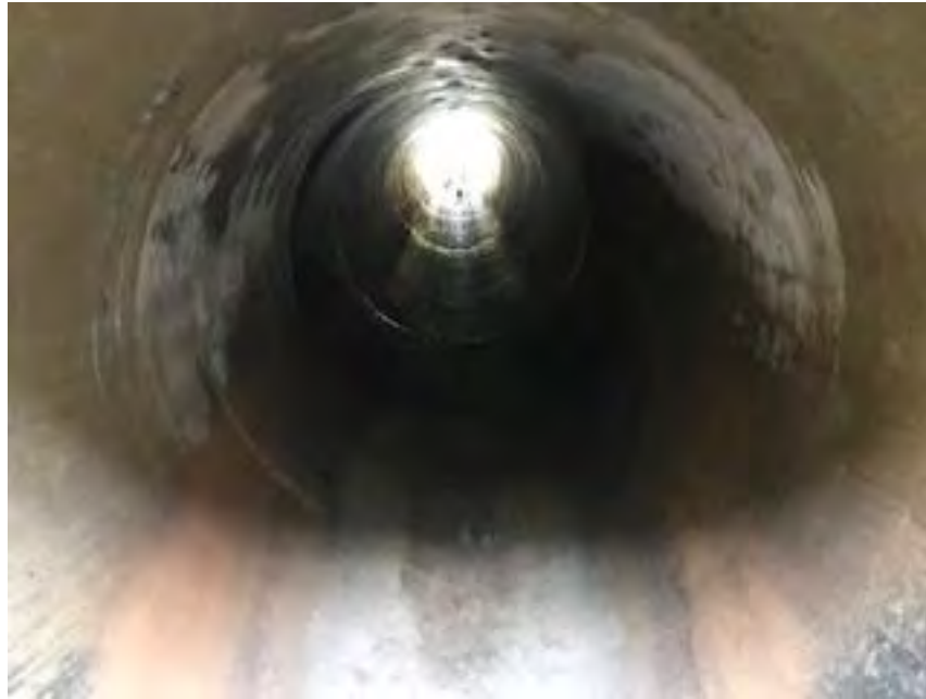
Picture 3. Interior of the 2.5 m diameter concrete Morning Glory outlet spillway
