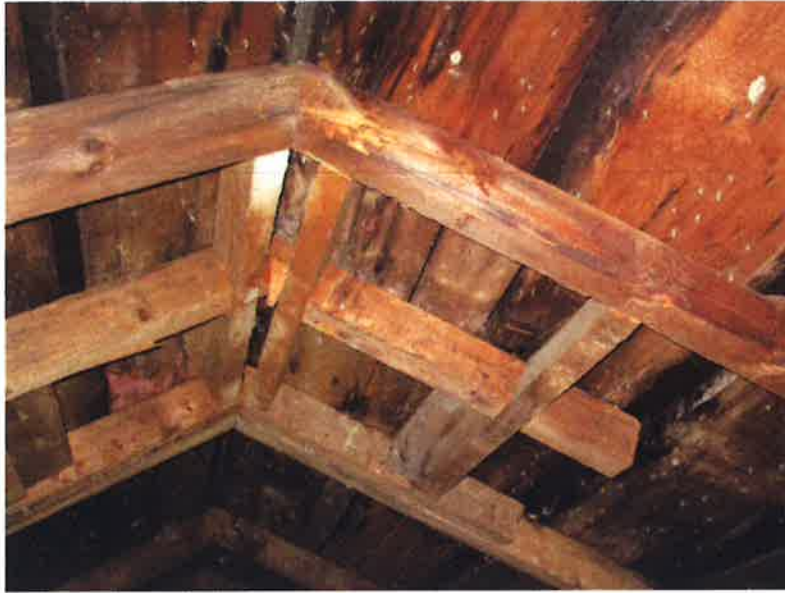
Roof infill at former chimney location
