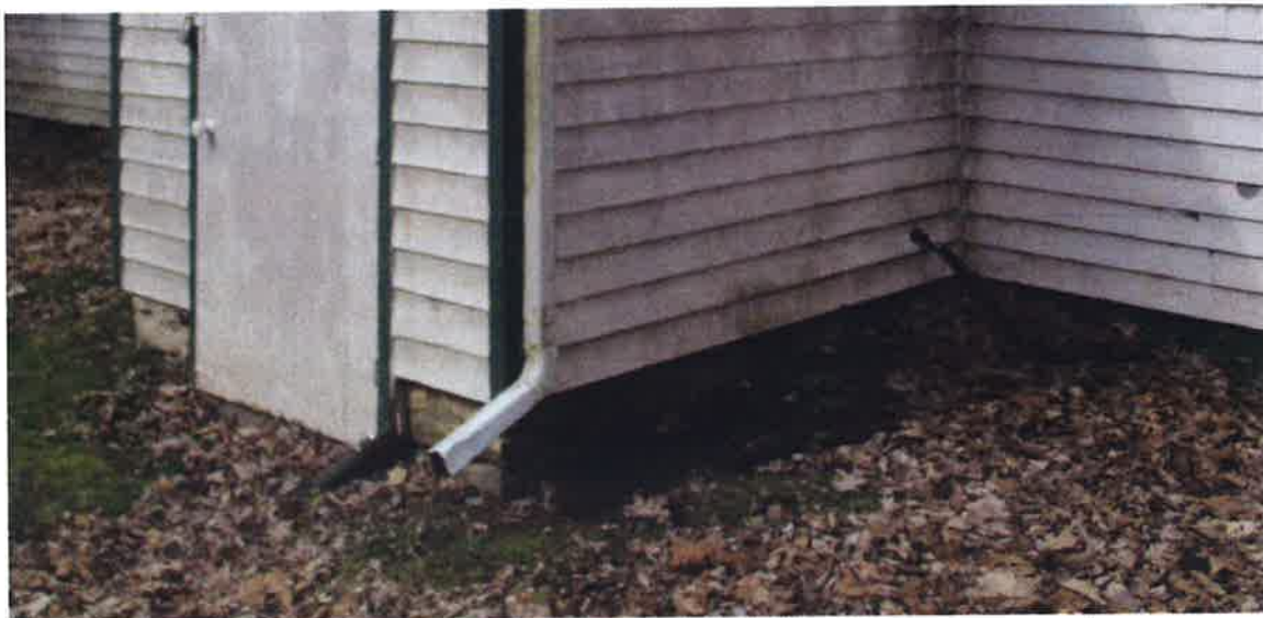
Sump pump lines and downspout discharging water on the east side
