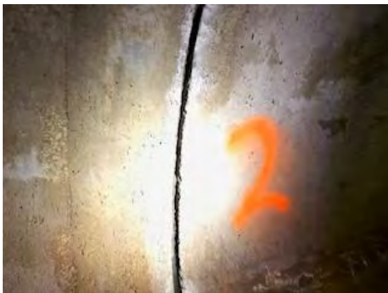
Picture 4. Joint cleaned of old sealant.
