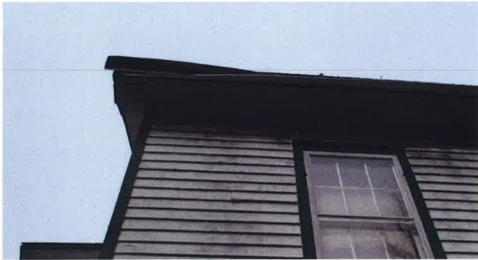
Eavestrough requiring repair
