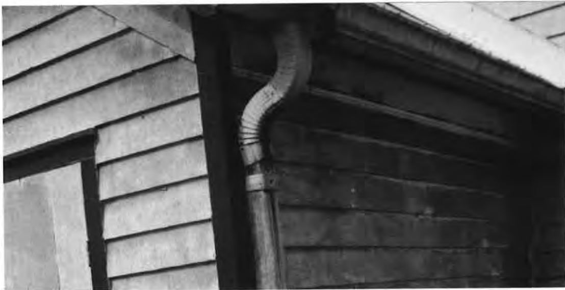
Downspout requiring repair
