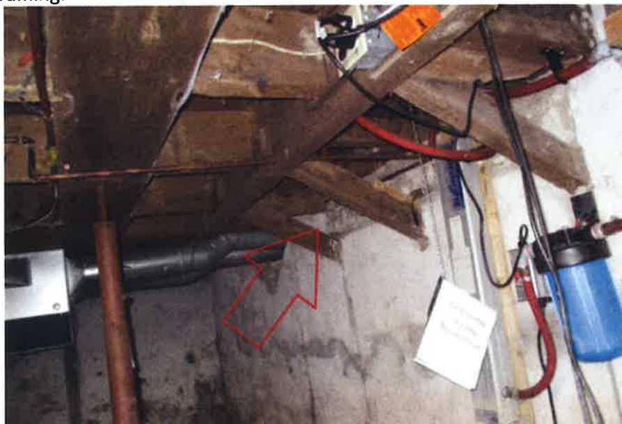
Ground floor framing at former fireplace location
