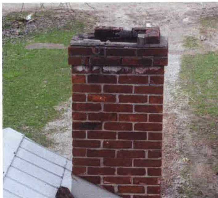
Kitchen chimney requires repairs and a cap
