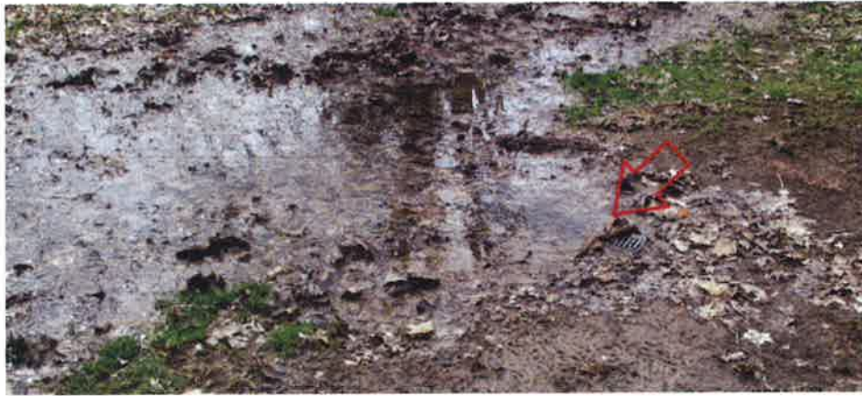
Sump discharge pooling uphill from the house
