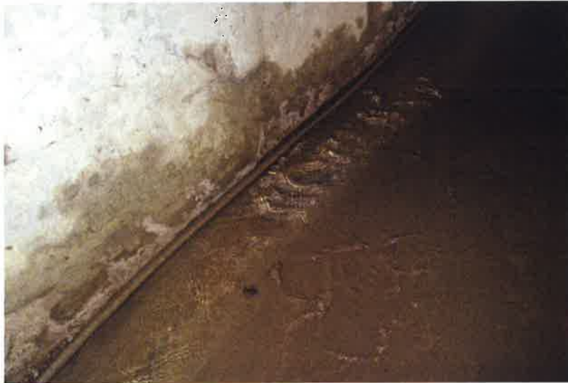
Water flowing across the basement floor
