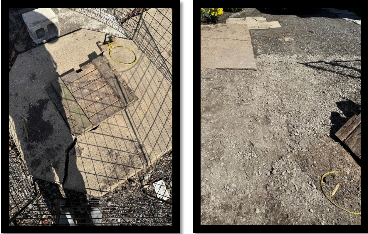
Figure 23: Before and after photos from a water well decommissioning project.
