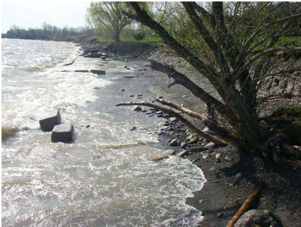
Figure 6.13 Ineffective Concrete Blocks (east of Hunter Road at boundary Reaches 1 and 2)
