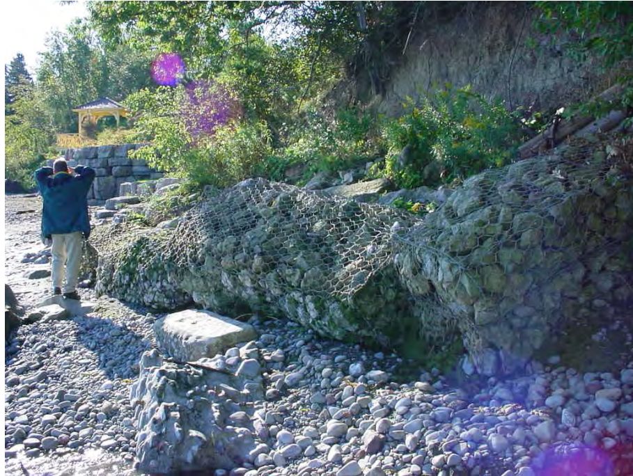
Figure 6.14 Collapsed Gabion Basket Wall
