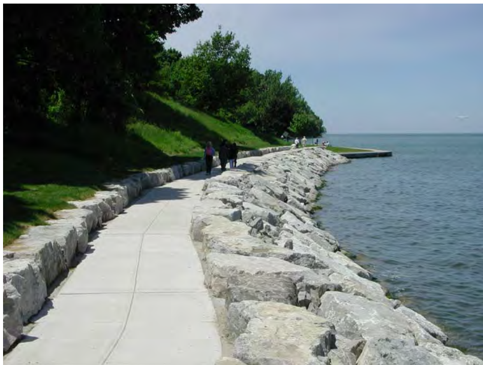
Figure 6.2 Armour Stone Revetment (Queens Royal Park, NOTL, Reach 5, constructed 2004)
