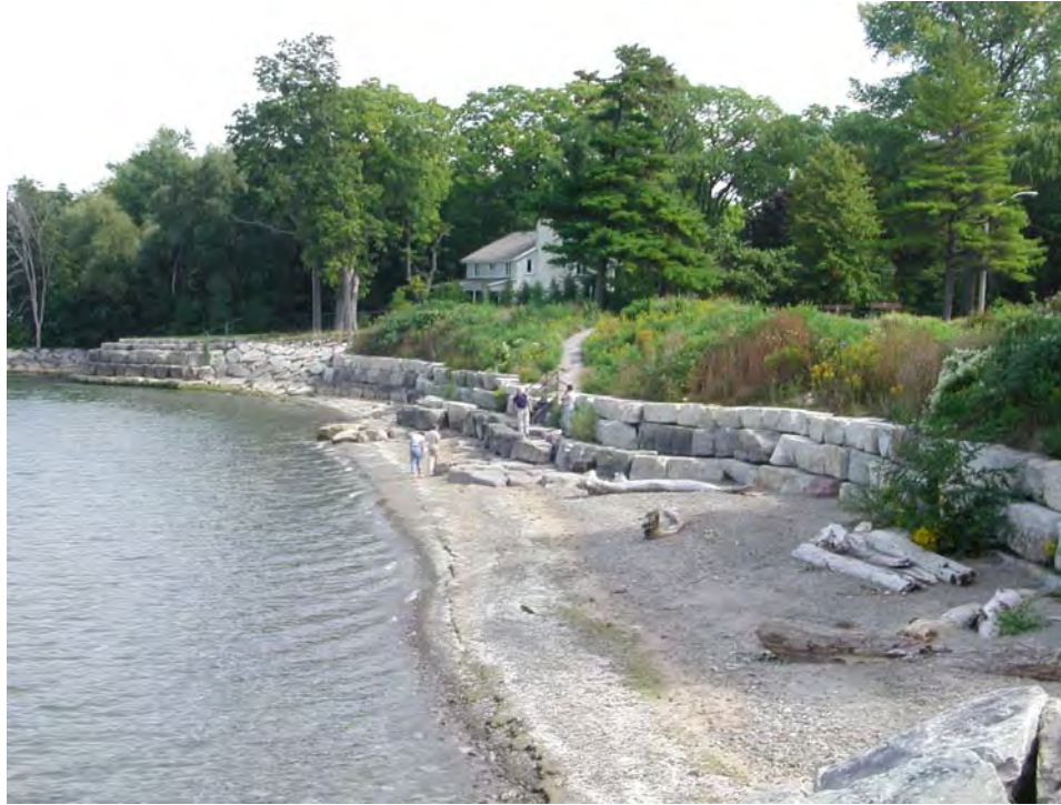
Figure 6.10 Stacked Armour Stone Wall (Ryerson Park, NOTL, Reach 54; constructed 1997)
