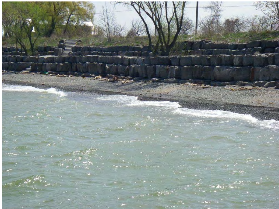
Figure 6.11 Stacked Armour Stone Wall (Site 11 east of Bartlett Ave; Reach 12; constructed since 2006)
