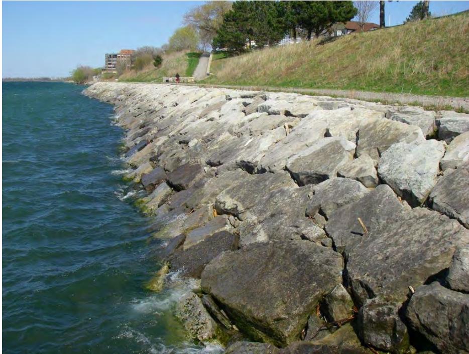
Figure 6.1 Armour Stone Revetment (Belmont Park at Beachview Drive; Site 26, Reach 22)
