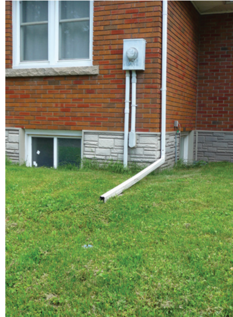
Disconnected downspout Kerry Royer, photographer
