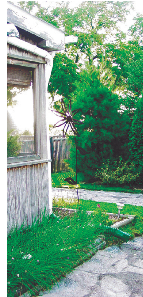
Disconnected downspout Jocelyn Baker, photographer
