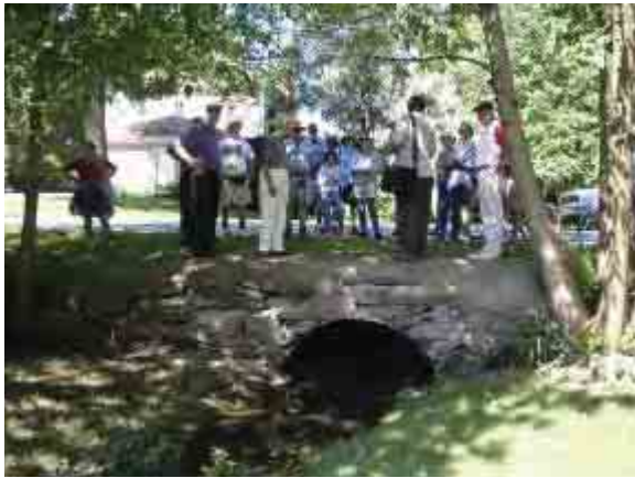
Zone 2 – Undersized Culvert
