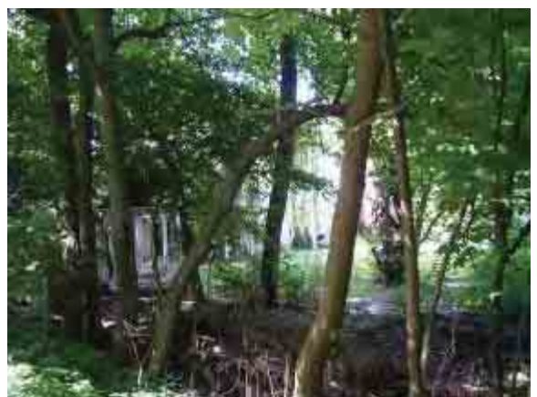
Zone 2 – flood susceptible structure
