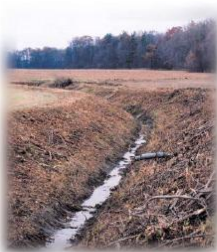
Brushing leaves the root systems intact, stabilizing the banks from erosion. Debris from the brushing protects the banks from wind and rain erosion.
