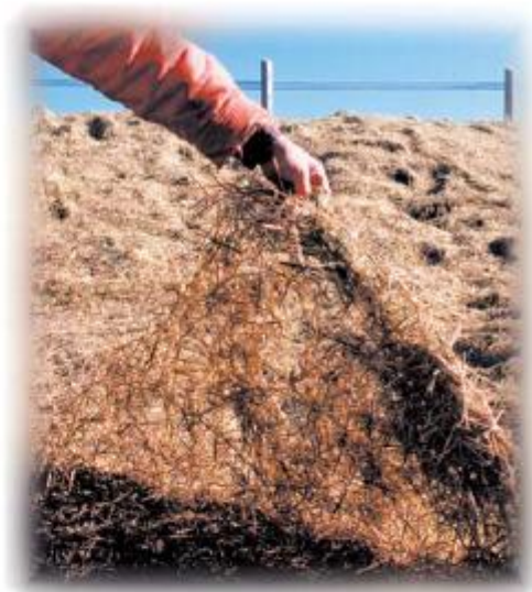
Straw blankets, such as the one seen above, help protect the exposed area from wind and rain erosion, and incorporate natural materials to help vegetation get reestablished.
