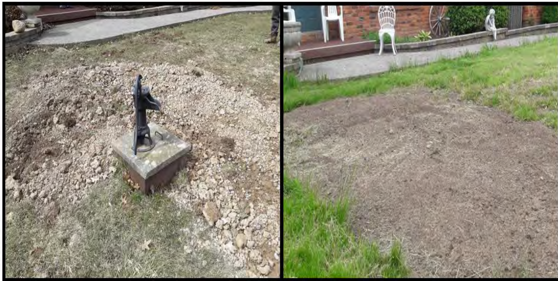
Figure 12: An example of a NPCA Water Well Decommissioning Project. Left photo shows an abandoned drilled well in need of decommissioning and the right photo shows same well after decommissioning had been completed by a licensed well contractor.
