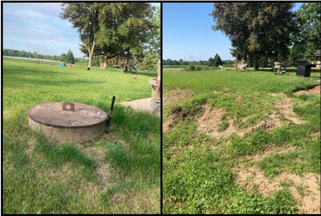
Figure 12: An example of a NPCA Water Well Decommissioning Project. Left photo shows an abandoned dug well in need of decommissioning and the right photo shows same well after decommissioning had been completed by a licensed well contractor.
