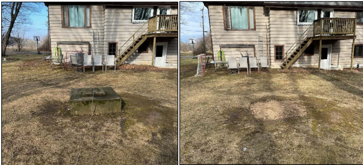
Figure 14: Before and after photos from a water well decommissioning project.
